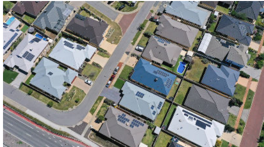
Roughly one in every three Australian homes now has solar panels. (Supplied: Project Symphony)
