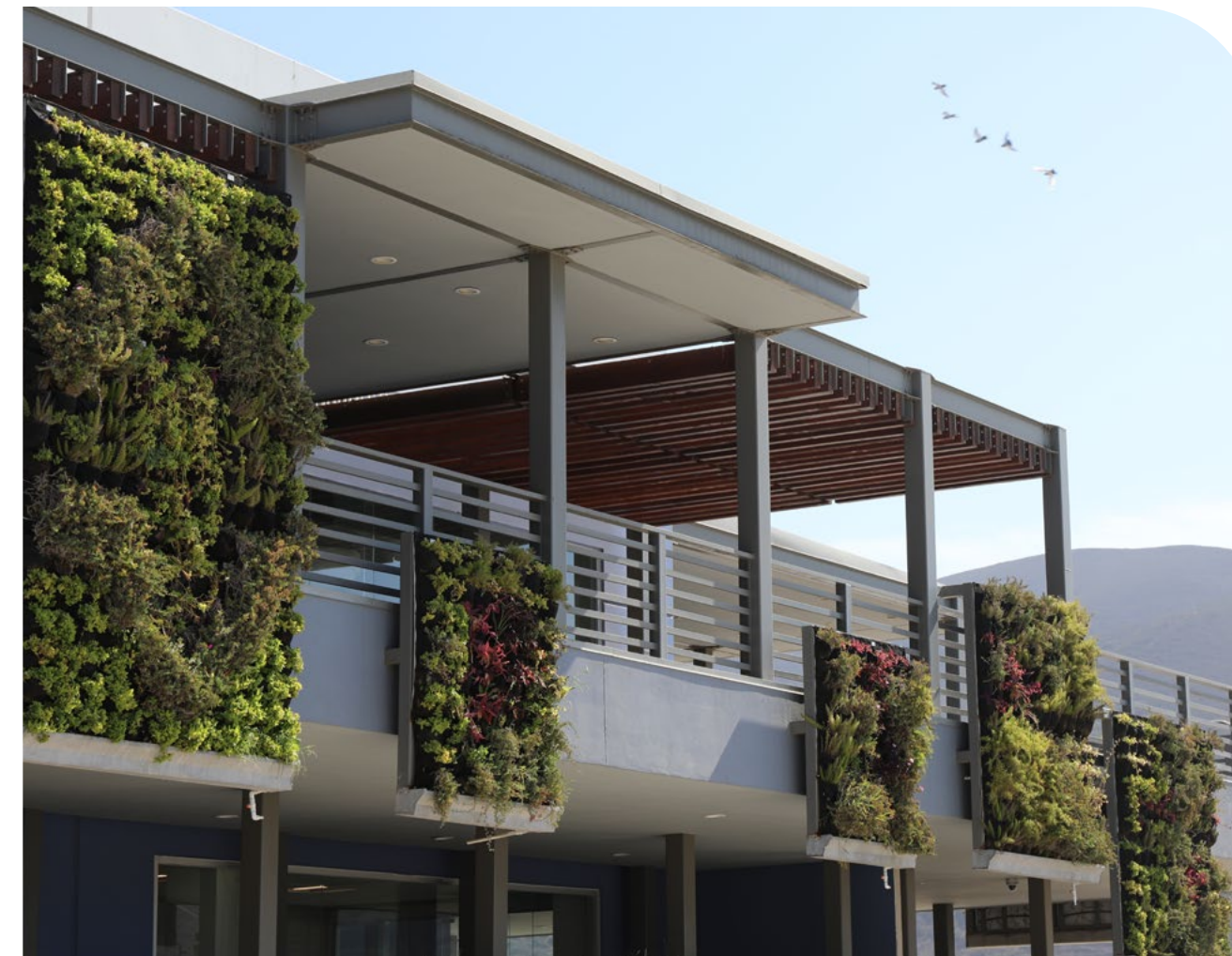
Ensenada, Mexico MODCO facility
