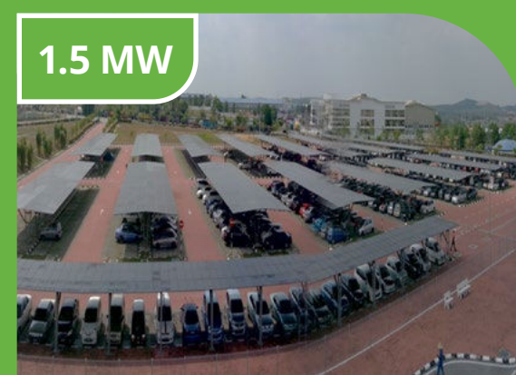
3. Covered carpark and motorcycle area
