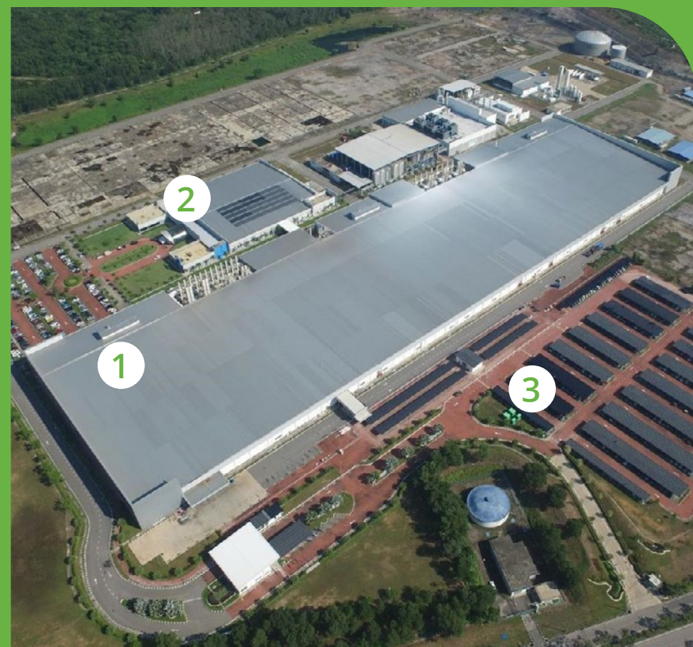
1. Future planned – FAB rooftop
