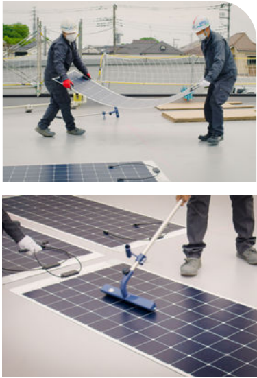
Installation of Maxeon Air solar panels
