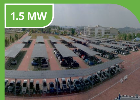
3. Covered carpark and motorcycle area
