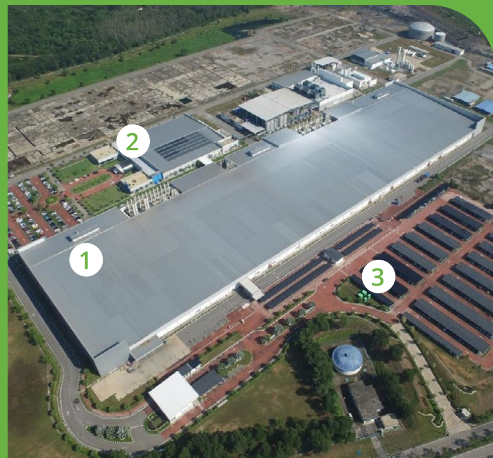
1. Future planned – FAB rooftop
