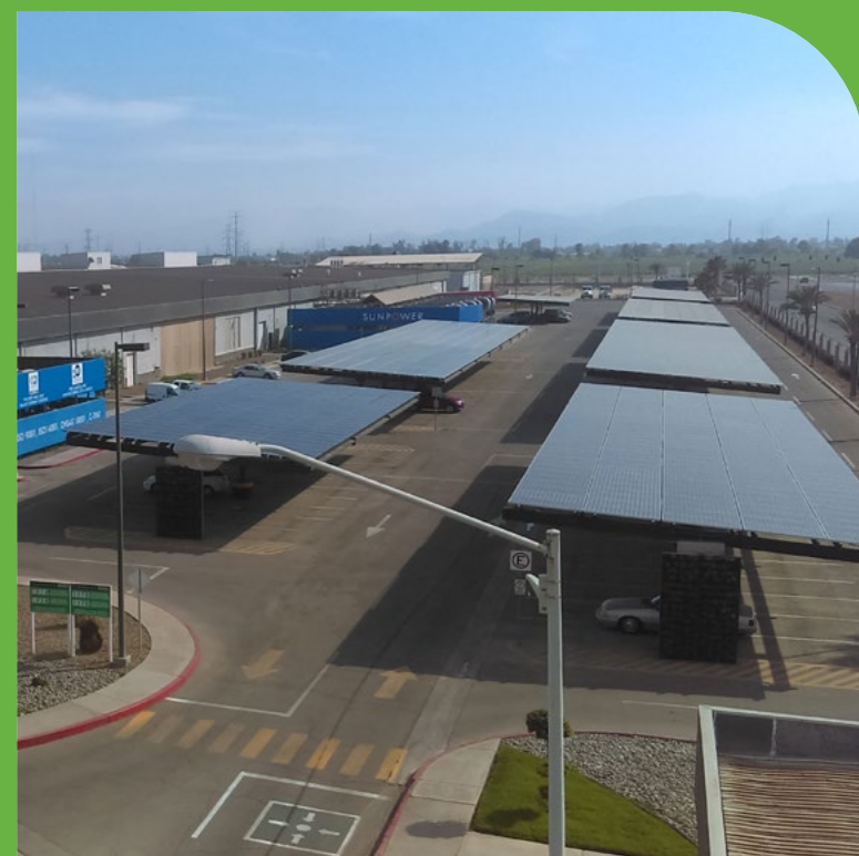
Solar panels installed as part of our carport project in our Mexicali plant (SPMX1)
