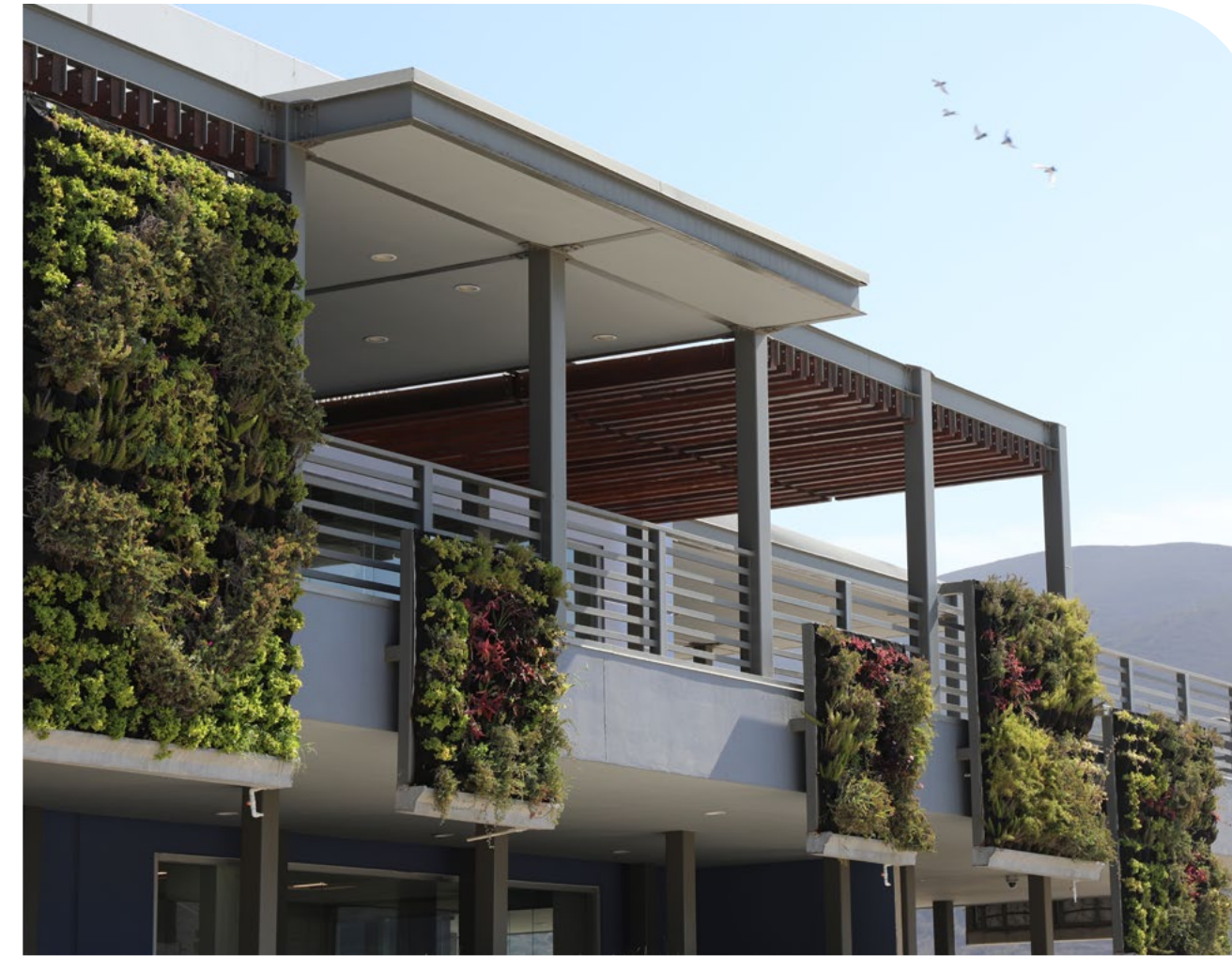
Ensenada, Mexico MODCO facility
