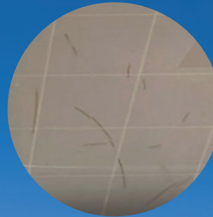
Widespread backsheet cracking PVDF
