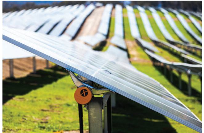
Having a hail stow mechanism can help reduce panel damage during hail storms. Image: Nextracker
