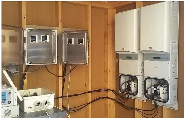
Figure 3.2.2 Power electronics and monitoring equipment
